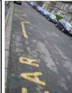
Carriageway south of Evelina Rd
